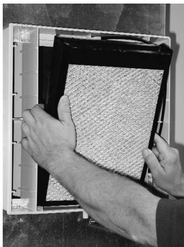
STEP 3: Clean or replace scale control insert. Replace Water Panel
